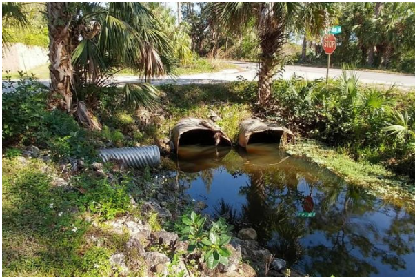
Figure 14. Canal Culvert under 175th
