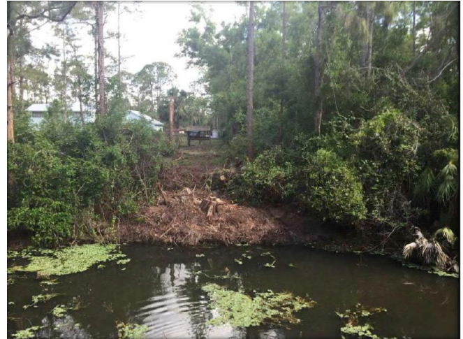
Figure 13. Needed Slope Repair
